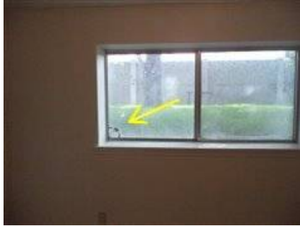
Photo 56-2 Basement, North end, East facing
