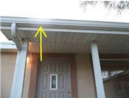
Photo 10-1 West side of home
