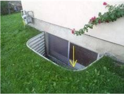
Photo 4-1 West side of home
