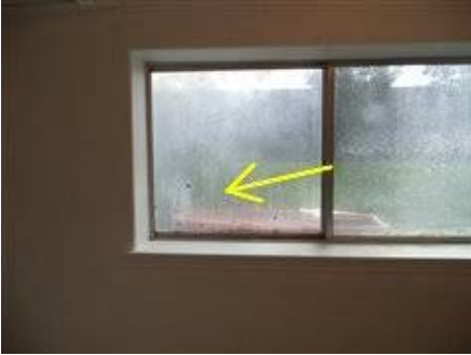
Photo 56-1 Basement, East facing
