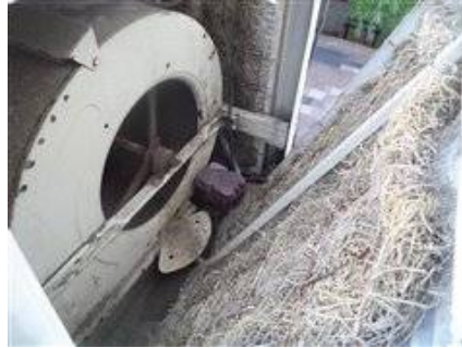
Photo 35-2 Roof, Interior of evaporative cooler
