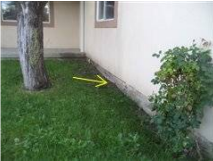
Photo 7-1 West side of home
