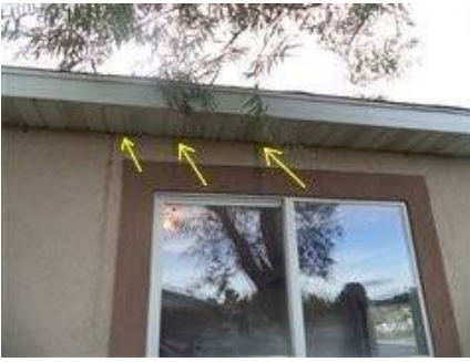
Photo 6-1 West side of home
