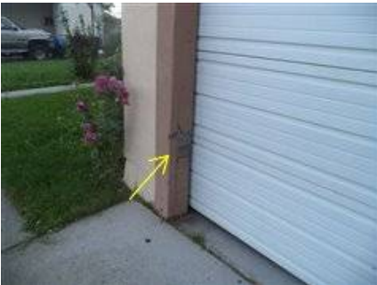
Photo 5-1 West side of home
