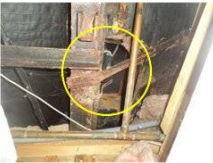
Photo 42-1 Basement, Under main floor bathroom
